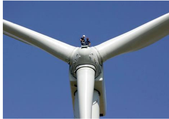
Wind turbine blades joined by bolts to the hub
